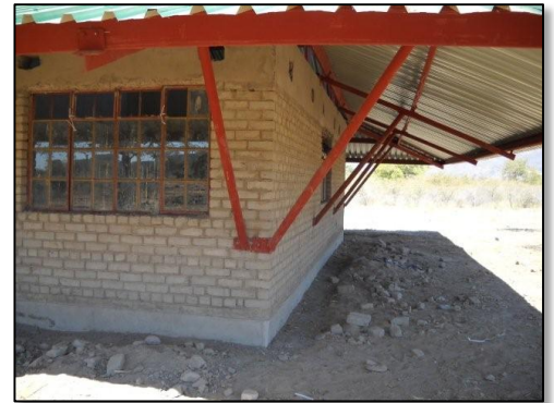
Windows going in
