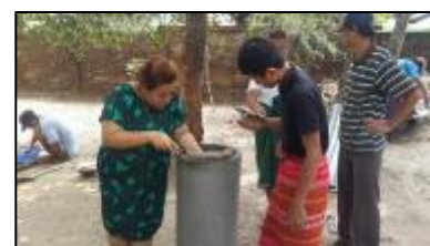
Working on the cement filters
